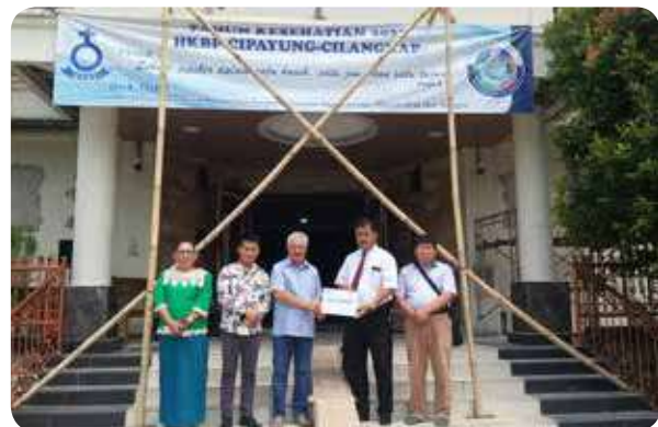
▶ Perbaikan gedung gereja di Cipayung Renovated a church in Cipayung
